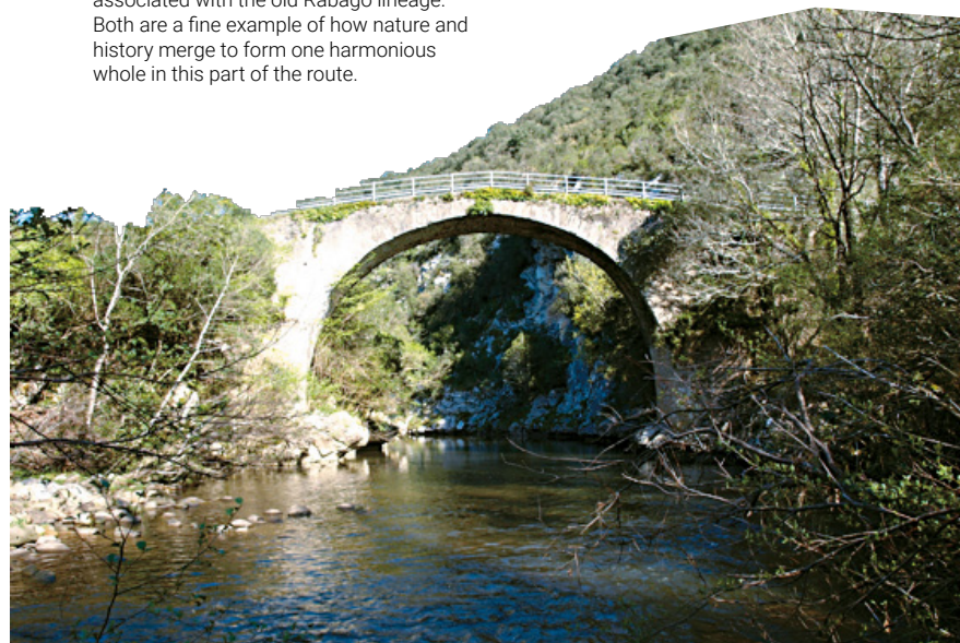
Tortorio bridge over the Nansa river ▶
