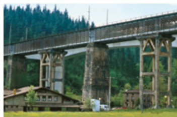
Railway viaduct, Ormaiztegui
